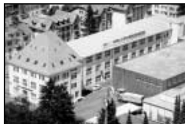
Hardinge Kellenberger facility St. Gallen, Switzerland
