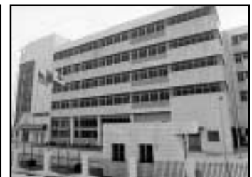
Hardinge Shanghai facility People's Republic of China
